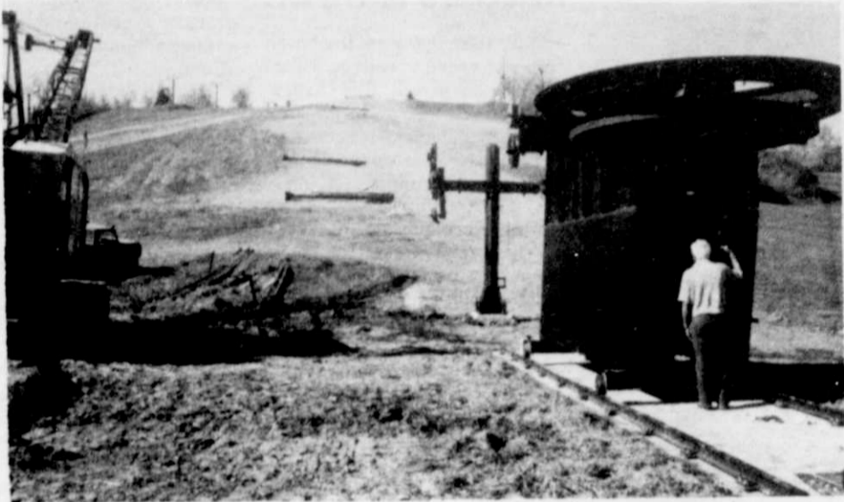
Sunburst employees worked on the power unit of the new chairlift.
