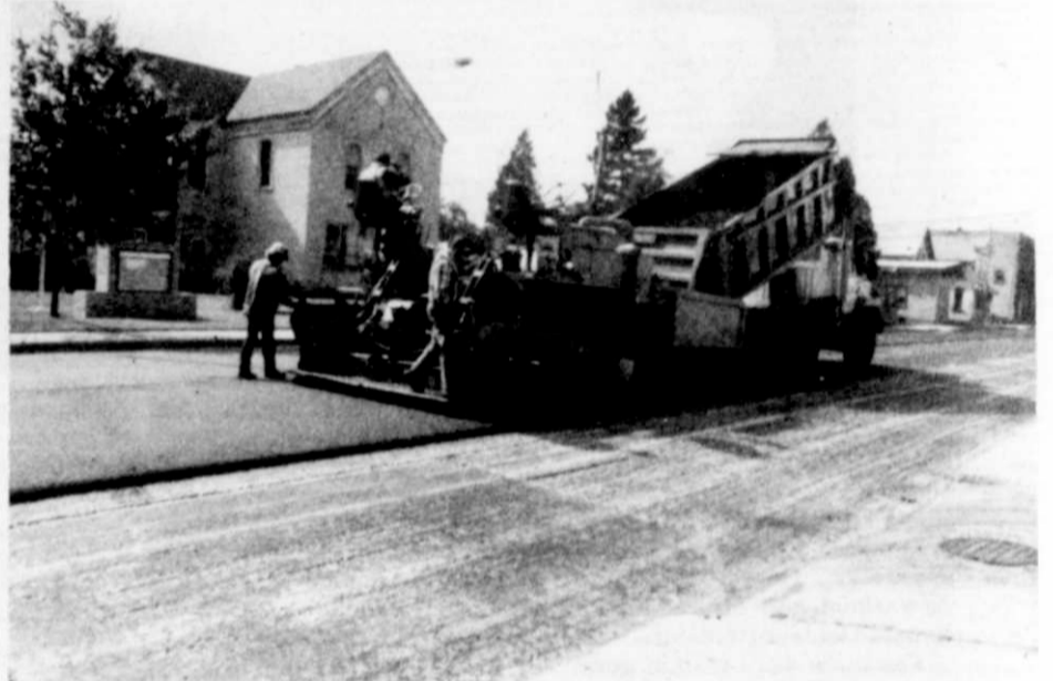
Tons of asphalt churned out daily were hauled to the paving machine as it slowly made its way down the prepared roadbed laying a thick black ribbon of blacktop along Main Street.
