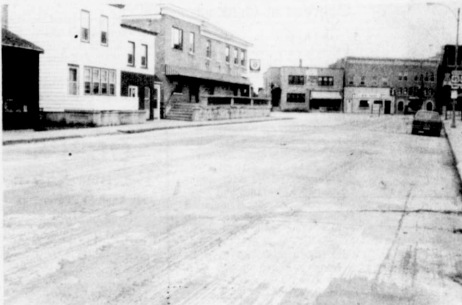
Desolate and forlorn looking, Main Street was deserted except for one lone car as it waited for its new coat of asphalt.
