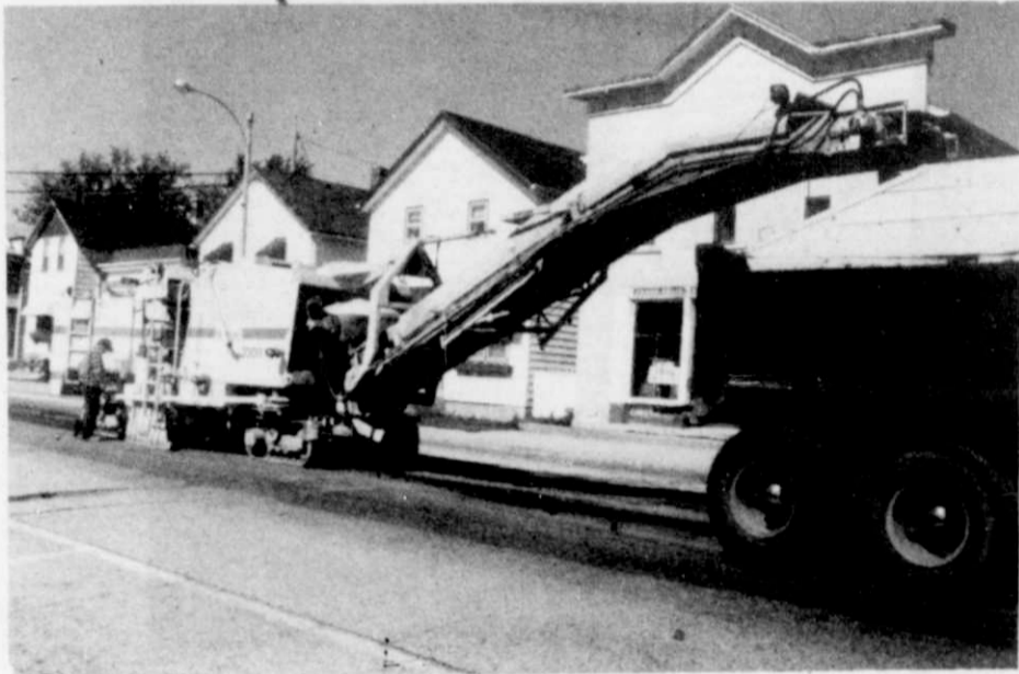
It chops it up, scoops it up and dumps it into a truck to be taken to the portable asphalt plant where it is recycled with new materials for the repaving process.
