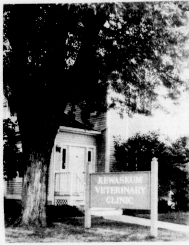
The new home of Kewaskum Veterinary Clinic on Fond du Lac Avenue.
