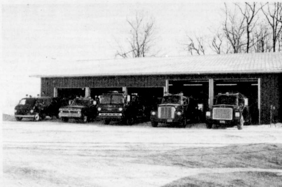
The Beechwood Fire Department moved into their new quarters on Saturday. The new garage has five bays and approximately one-third more space than the old firehouse that they had occupied since 1961.
