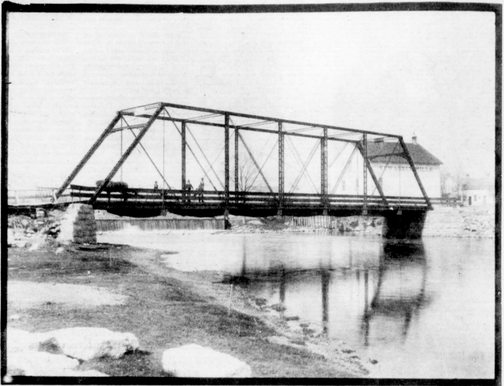
The old iron bridge over the Milwaukee River was believed to have been built in the early 1880's. Note the mill race (a canal in which water flows to and from a mill wheel), and the mill at the right. The dam is in the background on the left.
