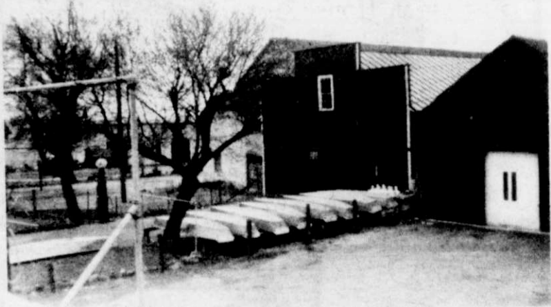
This photo was taken in the spring of 1939 at H. Ramthun & Son Boat Builders. It shows some of the metal boats manufactured in their machine shed at the rear of their hardware store on Fond du Lac Avenue.
