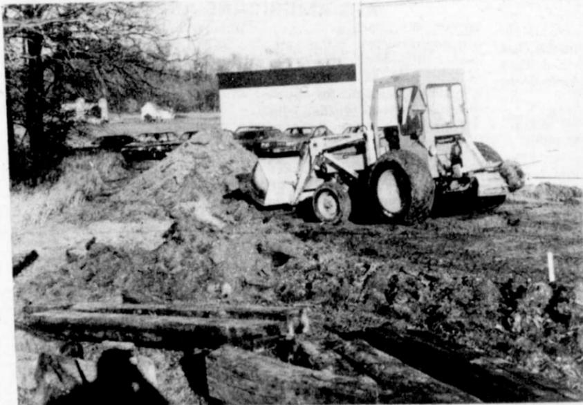
Initial construction of the driveway was accomplished with the use of the school's tractor. Here the sod is being scraped out to get down to a soil base.
