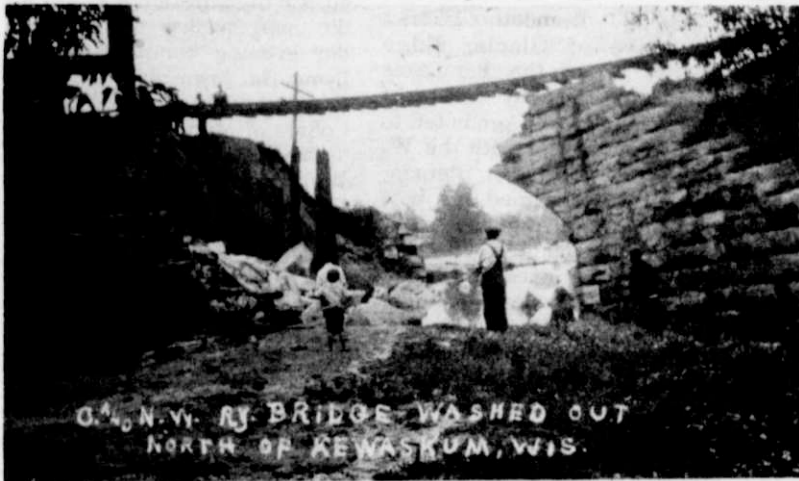
Washed out railroad bridge near north village limits in back of Herbert Backhaus and Julius Dreher homes on Fond du Lac Ave. Photo was taken two days after flood when water had subsided.
