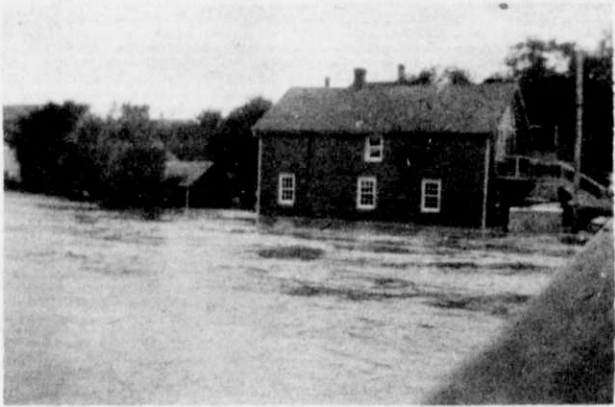
High water on the Milwaukee River at the Otto "Colonel" Stark blacksmith shop on Main Street.
