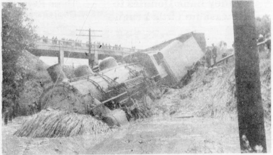
Train wrecked as a result of the washout from the flood near overhead bridge just north of the village. Engine shown in the ditch.
