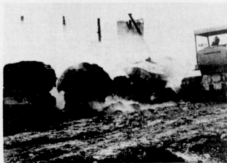
Smoldering bales and wall remains.
