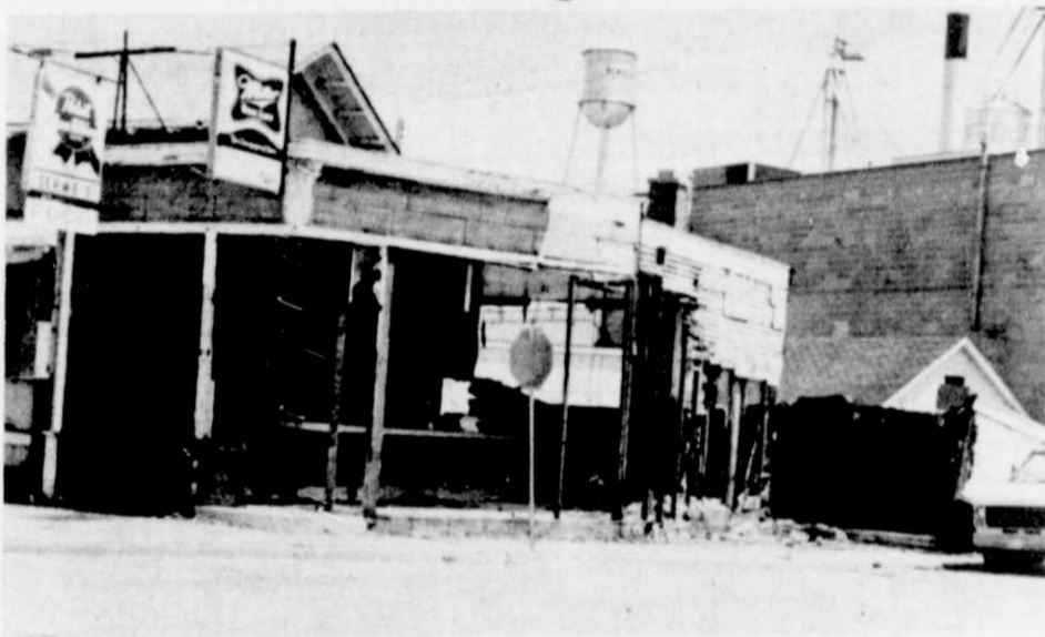
The tavern building half torn down.
