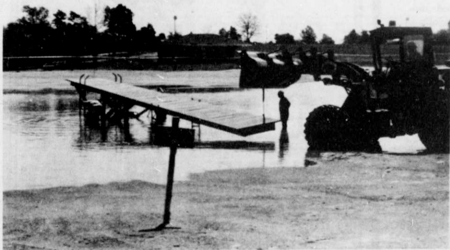
Another view of the pier
