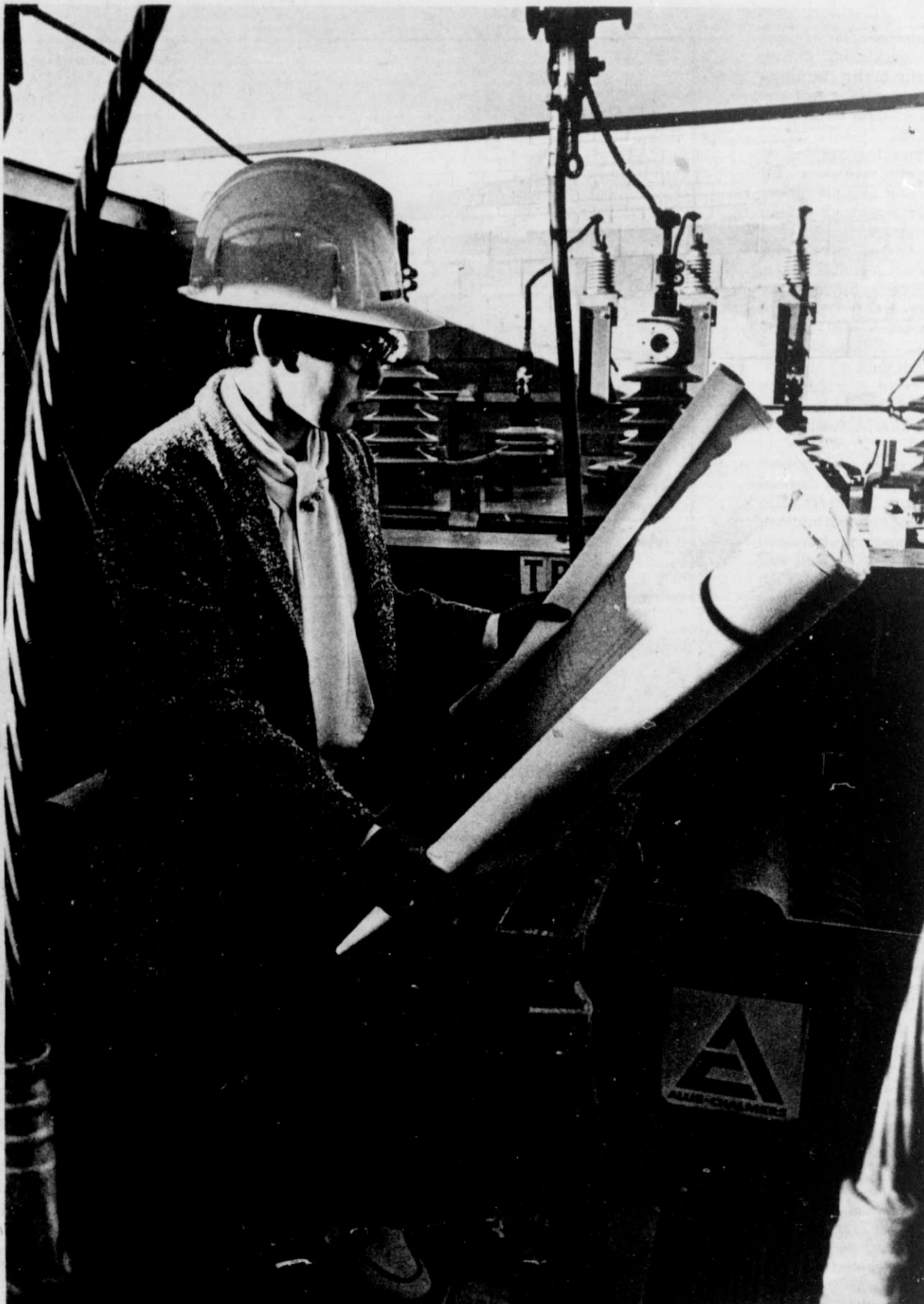
Kathy Young, senior electrical engineering technician at Wisconsin Electric Power Co., designed the utility's new Pike Lake Substation. Prior to startup of the facility, she checked over the equipment which will bolster the electricity supply in the Hartford, Wis., area. [Wisconsin Electric photo, December 1980]
