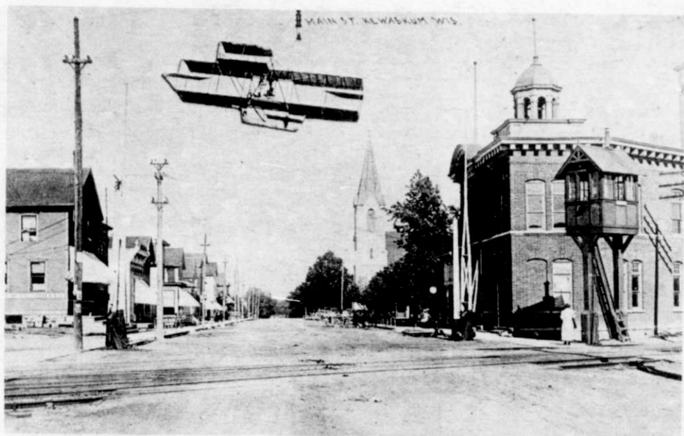
Here's another old picture of Kewaskum's Main Street east of the railroad tracks, dated 1914. Note the unpaved street, railroad crossing gates, signalman's tower on the right from where the gates were operated, the old village hall on the right with the fire alarm bell in the tower [now the Czaja building], and the old hotel building on the left which has been remodeled and is now Flynn's Bar.
