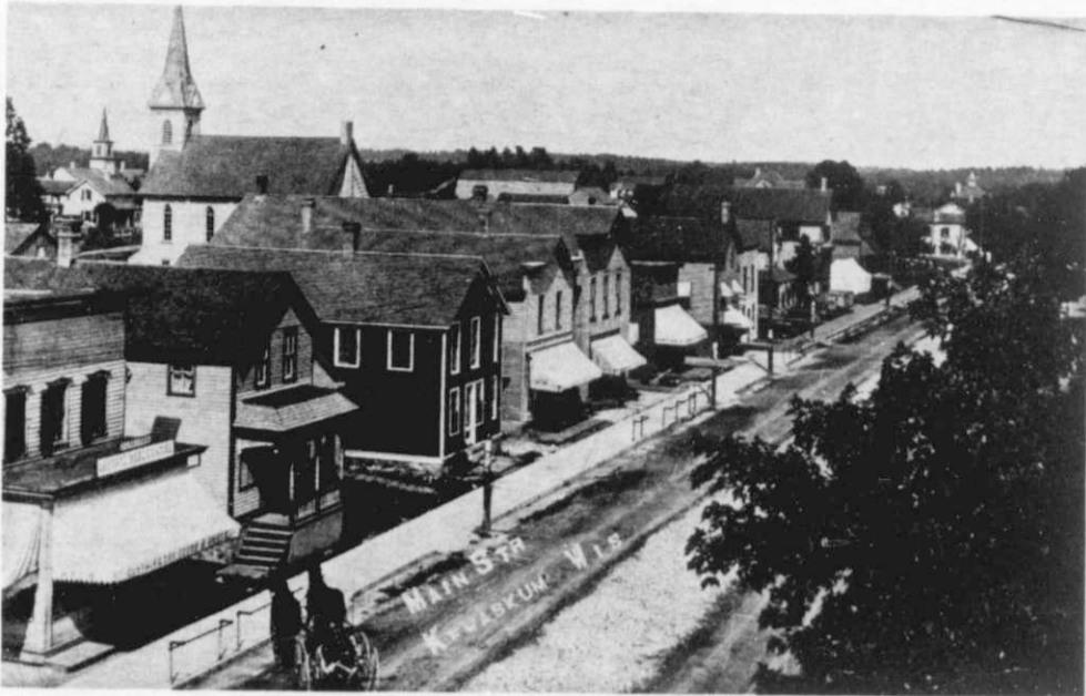
A picture of the north side of Kewaskum's Main Street east of the railroad tracks, taken about 1913. Note the Peace and St. Lucas churches in the background.
