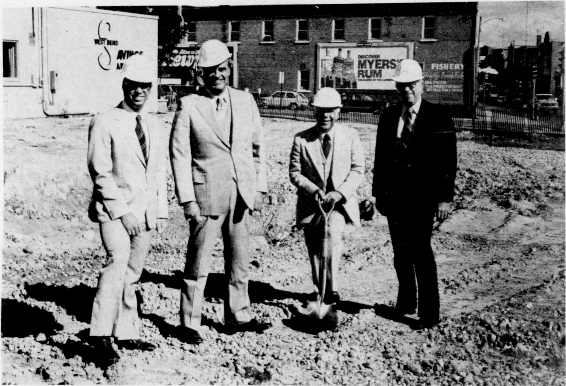
Pictured from left to right: City Centro President John Torinus; Mayor John Pick; West Bend Savings and Loan President Richard Larson; and Allyn Raymond, president of Bank Building Central, construction supervisors.
