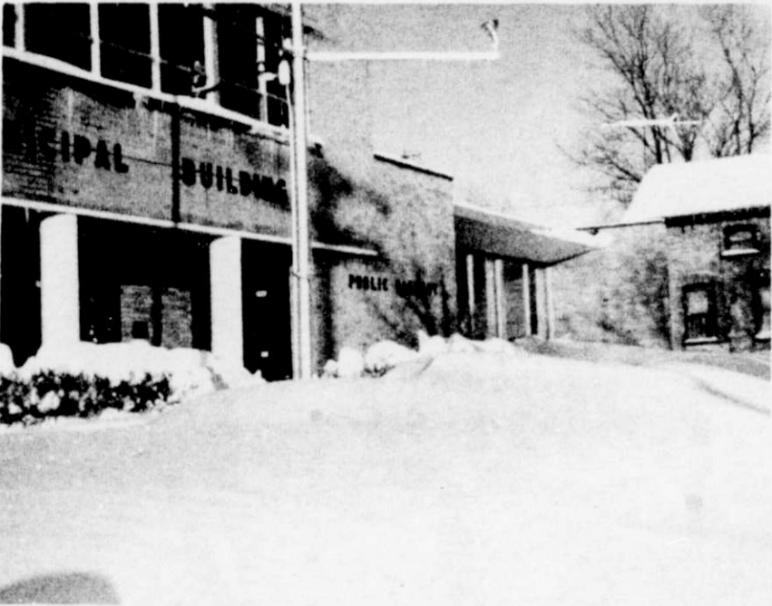
Snowbanks in front of the municipal building.
