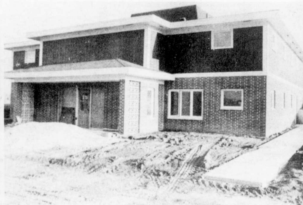
March 3 issue — Tuesday, Feb. 28, marked the opening day of the Sison Professional Building at 1040 Fond du Lac Avenue in Kewaskum. The building is shared by Drs. Cesar and Aurora Sison, Dr. Florizel Castro, Drs. Renato and A. Estrella, Dr. Dennis Connor, D.D.S., the staff and a pharmacy.
