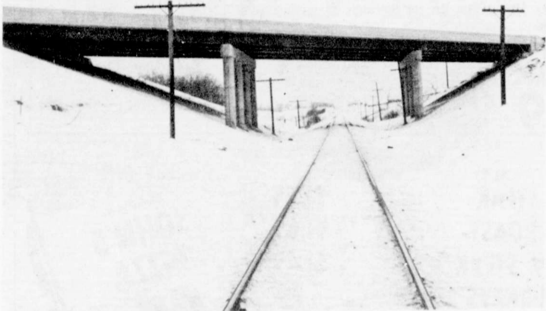
The new Hwy. 45 overhead bridge at the north village limits.
