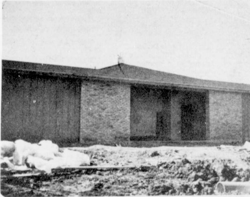
Front view of the bathhouse
