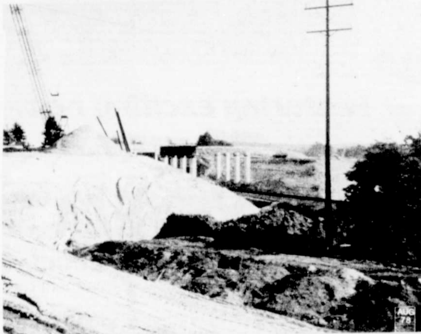
The above photo was taken in August with two of the piers and some of the grading completed and the abutments yet to build.
