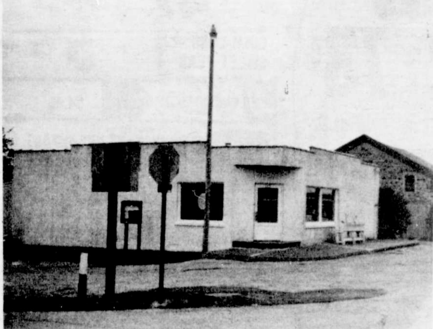
The present building which was completed in the spring of 1949.
