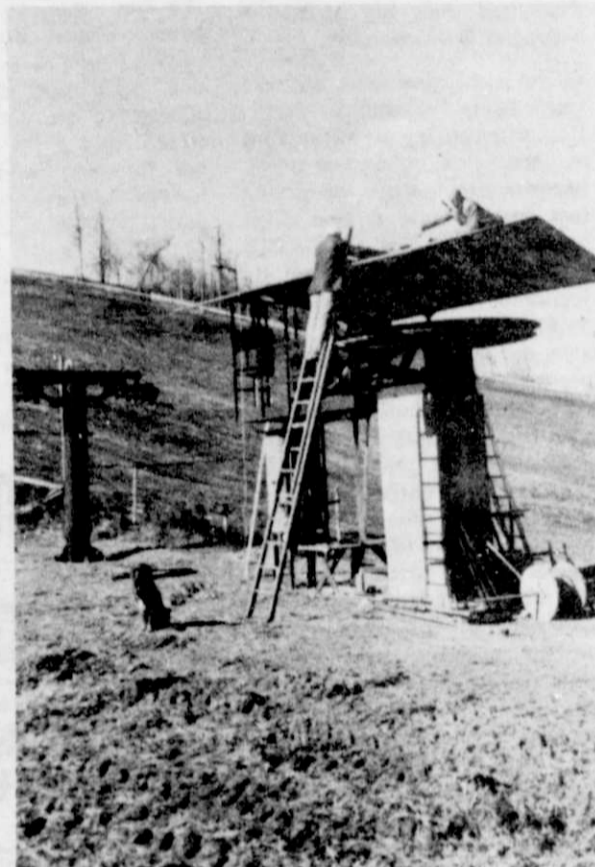
Construction of roof over bull wheel and motor.
