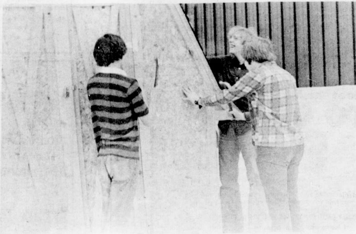
Students in the building trades course have constructed utility barns which are resold.
