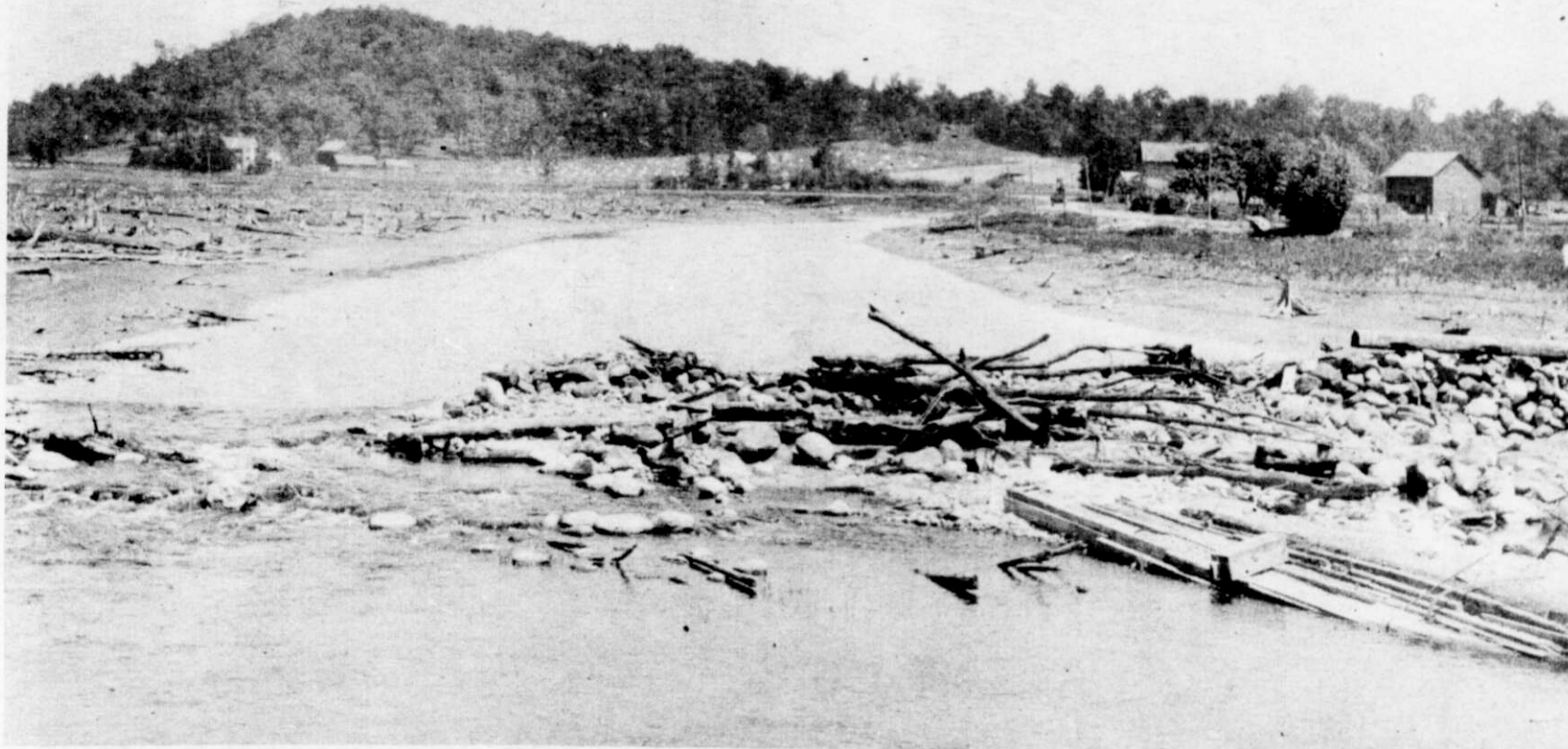
The old dam went out in 1911.
