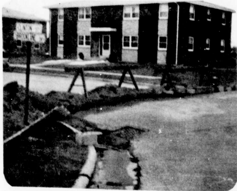
This barricade was set up by village crews at the corner of Brooklane Dr. & Clinton St. to divert the water to the creek at the south end of the village after Friday
