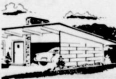
and eight feet long, between 4 by 4-inch posts set into the concrete driveway. Readily pliable for this weaving process, the Masonite siding is easy to work with, as it is splinter-free and free of defects. It takes a beautiful paint finish and will last for years.
