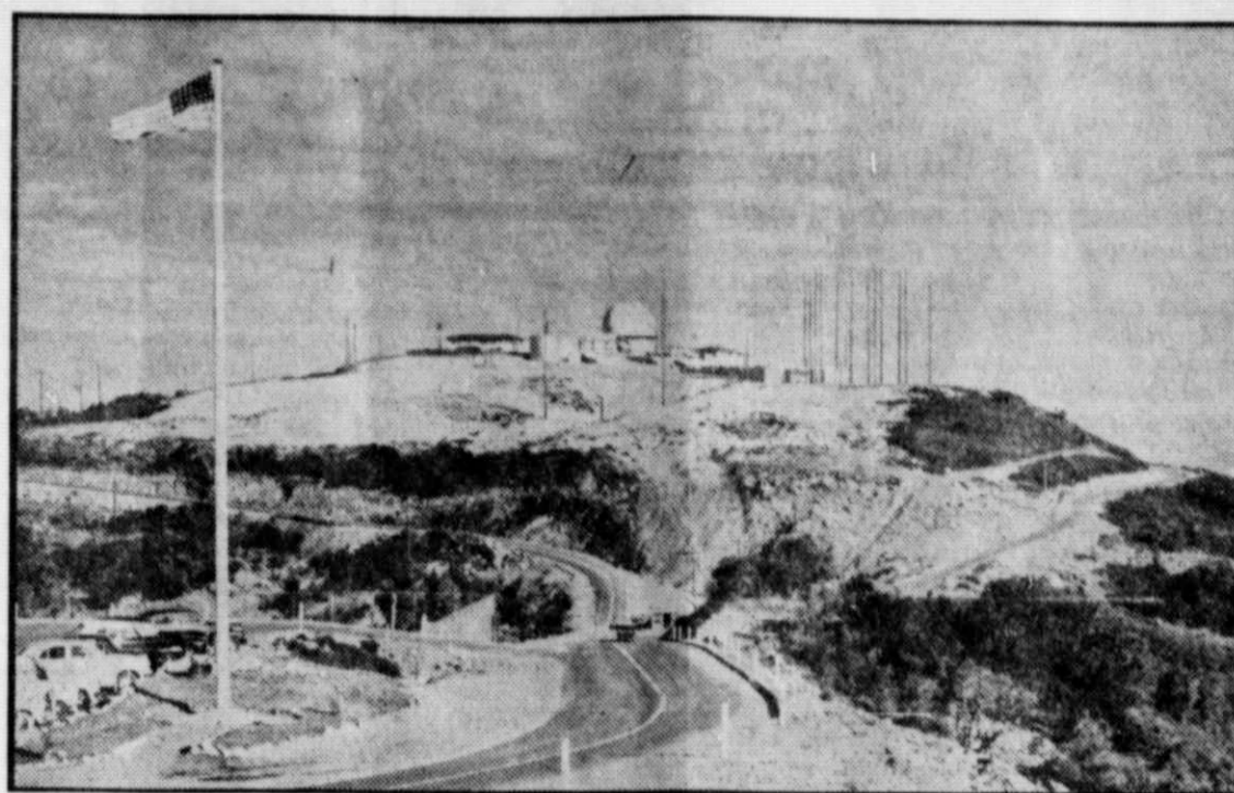
WATCHDOG MOUNTAIN — An "around-the-clock" sky watch is kept to guard the San Francisco Bay area from surprise air attack. The $5 million U. S. Air Force radar center on Mount Tamalpais picks up unidentified planes on radar screens and relays the information by radio to fighter headquarters at nearby Hamilton Field. The ball-shaped sphere at center stands 65 feet high and houses radar antennae. Wooden poles at right are 90-foot-high radio antennae towers.
