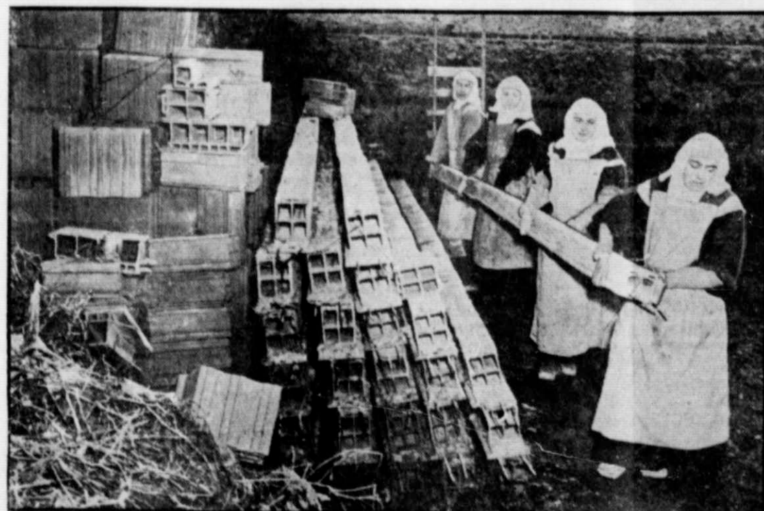
NUNS BUILD OWN CONVENT —Thirteen Carmelite nuns are building their own convent near Turin, Italy, with material donated by local parishioners. Here four of the nuns who will inhabit the convent are shown carrying a heavy cement base. When the convent is completed, the nuns, who took lessons from masons for two months prior to beginning work on the project, will retire to a life of cloistered silence.
