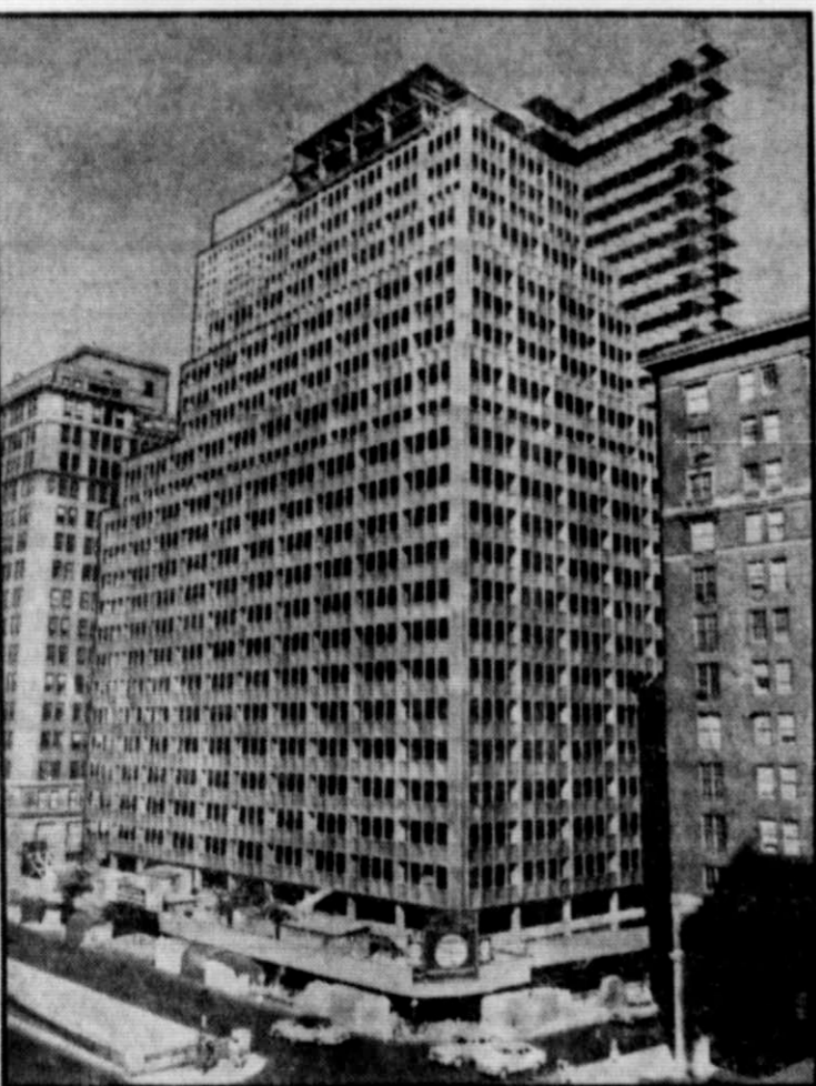
THIS AGE OF SPEED—Latest addition to New York's Park Avenue skyscrapers donned its prefabricated skin in a record-breaking six-and-one-half working days. Three specially trained crews clad the 26-story skeleton of steel and concrete with 1800 prefabricated aluminum panels. Each panel contains two six-foot windows which rotate for safe interior cleaning. Ordinary brick-and-stone construction would have necessitated eight weeks for completion.
