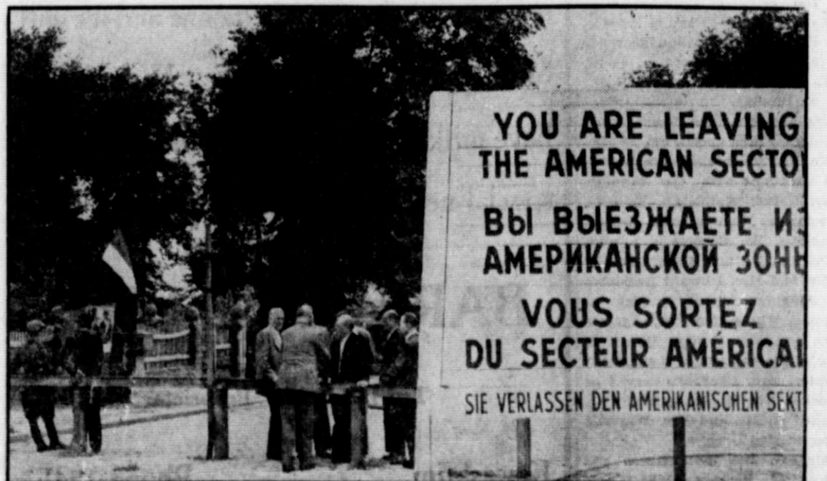
BRIDGING THE GAP—A severe water shortage in Berlin's Neukolin district momentarily washed away East-West barriers as officials from both sides met to discuss the problem. An earlier agreement on mutual water deliveries made possible this meeting on a bridge linking the American and Soviet sectors. Note East Berlin police "guarding" the meeting.
