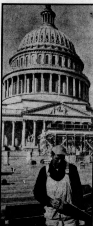
GETTIN' READY FOR IKE —Grandstands for the presidential inaugural ceremony are going up in Washington, will be done in time for use January 20. Washington carpenter, John Moore, saws seat boards. Seen in rear is the stand where Ike will take his oath of office.
