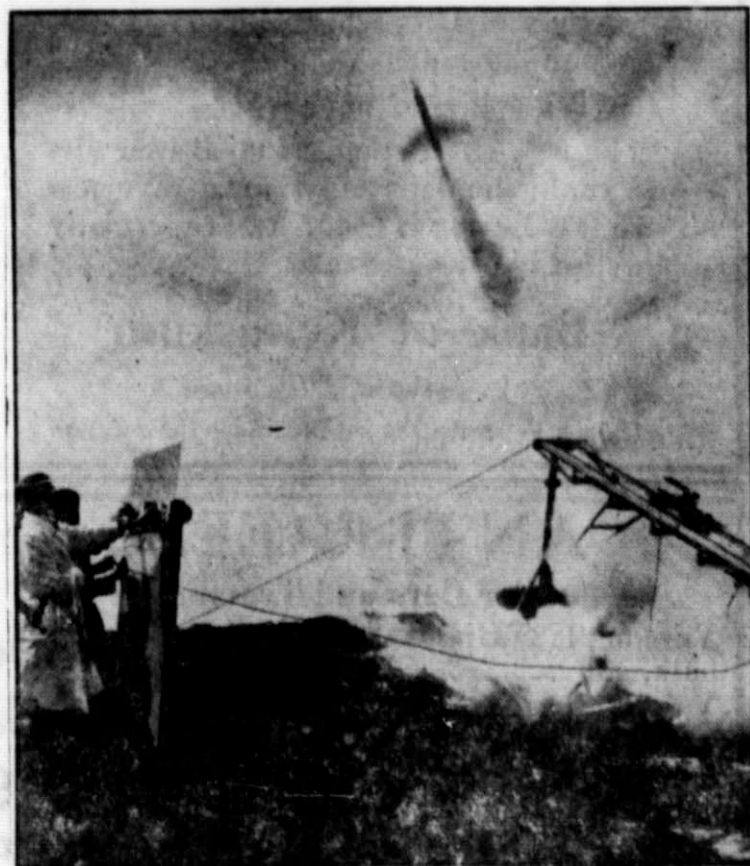
HIGH HOPES FOR ROCKET-MAIL—Prof. Albert Puellenburg, standing at switchboard on left, watches his rocket make the first of five test flights from a 20-foot ramp near Bremen, Germany. He is experimenting on mail-carrying possibilities of the missiles, using experience gained as designer of Germany's V-bombs which blasted London during World War II. Allied security inspectors watched the experiment and saw Germany's first postwar rocket in action.
