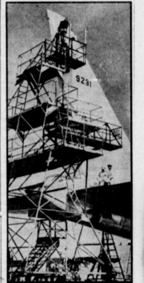
TALL TAIL—It's no tall tale when mechanics working on this highly secret eight-jet bomber in Seattle say the huge ship is "way up there" even when it's on the ground. Special scaffolding is needed to permit adjustments on the 48-foot-high vertical tail.
