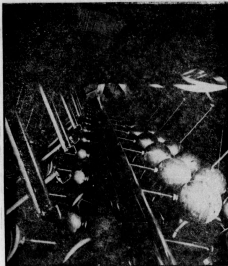
FOR A MULTI-VOLT JOLT —Capable of re-enacting Benjamin Franklin's famous kite, key and lightning experiment of two centuries ago, is this generator at General Electric's Pittsfield, Mass., laboratory. A worm's eye view shows the 50-foot-high lightning maker from this unique angle.
