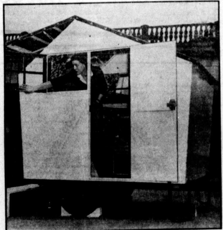
FOLDING HOUSE—One of the new features on display at the annual sports and camping show in Paris is this trailer-mounted folding house. Designed for rapid assembly, the camping hut is extra light for use with a small car. It houses three persons.
