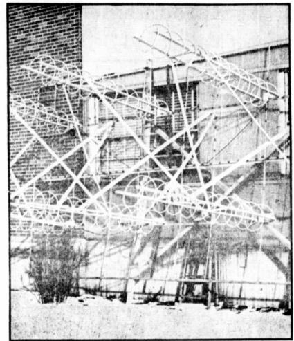
COLUMBUS LISTENING POST—The curlicue tubules jutting from the wall are parts of a radio-telescope designed by Dr. John Kraus of Ohio State University at Columbus. Dr. Kraus hopes to pick up radio signals from stars 1,000,000 light years away from the earth. He says the signals produce a "frying sound" on the
