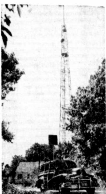
SUCCESS HILL—The lofty antenna of the Bridgeport UHF station towers over the white frame station house at the left. In the foreground is a station wagon equipped with UHF receiver and portable antenna. It has been used to test signal strength throughout the Bridgeport area. Station KC2XAK is the first and only UHF station in the country to operate on the regular daily basis. It is located on the crest of Success Hill on Bridgeport's outskirts.
