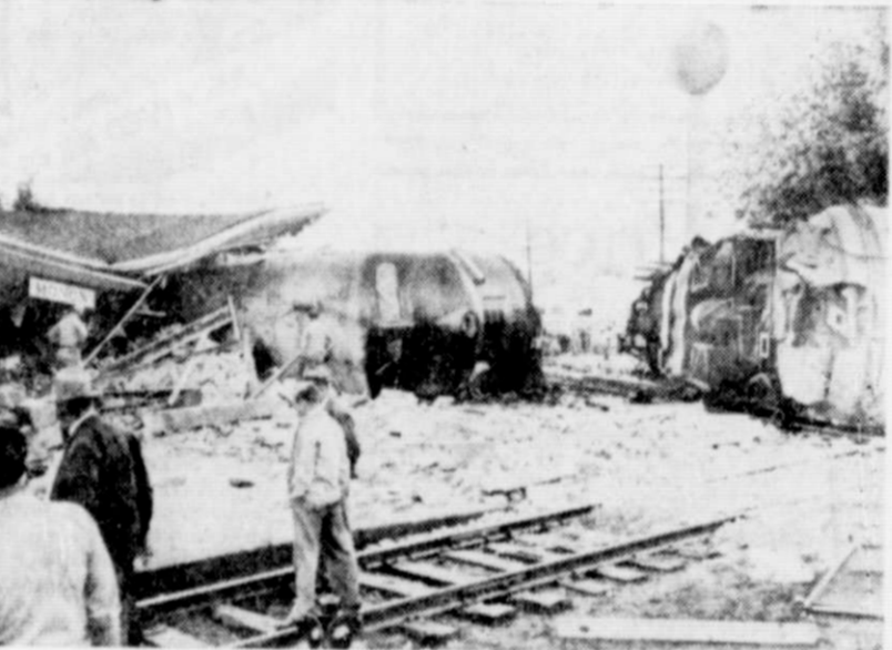
TRAIN DEMOLISHES DEPOT . . . Railroad officials are seeking the cause of a freak accident which recently killed one person and injured five others when a Monon railroad streamliner failed to take a curve and plowed into the center stone Monon railroad station. The ill-fated train was bound to Chicago from Louisville. Photo shows the demolished railroad station and the wreckage of two of the units of the diesel locomotive that pulled the fast streamliner before the wreck.
