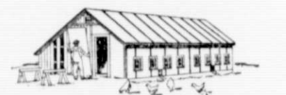
The building in the top picture is a discredit to any farm, while the one below, a remodeled version of the one above, will add to the farm's value.
