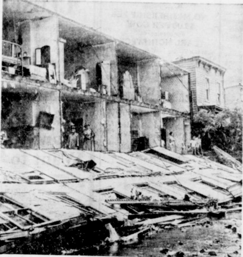
TORNADO DAMAGE . . . Amazed home-dwellers find themselves with plenty of air conditioning as a result of a 90-mile-an-hour tornado that ripped through Richmond, Virginia. At least 50 persons were injured, hundreds were left homeless, and property damage was estimated in the millions. House above was in 25-block section ripped by the tornado. The entire front wall of the two-story structure was neatly ripped off, producing house with a view.
