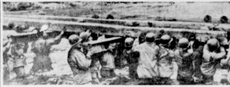
WET JOB . . . Engineers hoist girders across Korea's Hantan river.
