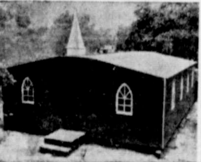
PORTABLE CHURCH... This portable Whittier, Cal., First Brethren church can be folded away like an accordion if necessary and carried anywhere by automobile. Complete with pews and pulpit, the church seats 120 persons.
