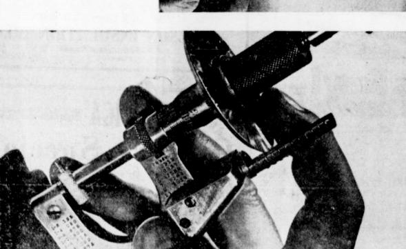
A standard 0-1.0-inch micrometer plus a simple vernier sliding bar and collar provide a means of measuring sizes accurately within 0.002 in. by touch. Raised lines on the vernier and the collar replace the usual numbers. The "mike" is set to the part to be measured and the size, to the nearest 0.025 inch, is determined by sliding vernier bar up against the lower edge of the knurl
