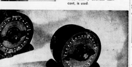
The instruments shown above are timing devices second-timers for blind people who work in photographic dark rooms. These instruments were developed after studies by the American Foundation for the Blind. At right is an outdoor braille thermometer, popular with blind poultry raisers and truck gardeners and for greenhouses. This product also is a result of research and development at the foundation for the blind.
