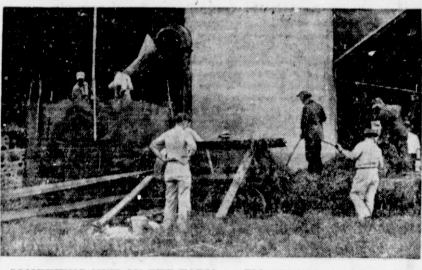
SOMETHING NEW ON THE FARM... This grass went to silage on a Wisconsin farm last summer. Temporary silo, made of welded woven wire covered with reinforced paper, keeps the silage in good condition.
