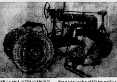
TILLS SOIL WITH 'GADGET' . . . For a total outlay of \$75 for welding and parts, James van Hyfte, 31-year-old farmer near Hillsdale, Ill., built this highly efficient, light weight tractor. A 1928 car engine is the heart of the tractor. A double transmission gives the machine six speeds forward and three reverse, making it adaptable to any kind of load, speed, field or road condition.
