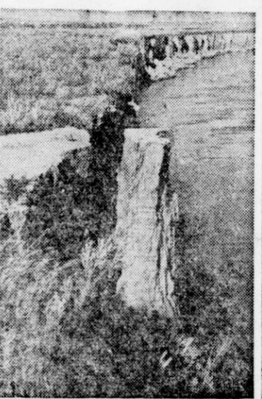
TOO MUCH WATER—The rampaging Missouri river is eroding millions of tons of good soil away every year. Here the flood waters carved into the bank, washing out a road, and leaving a pillar of earth to indicate the earlier line.
