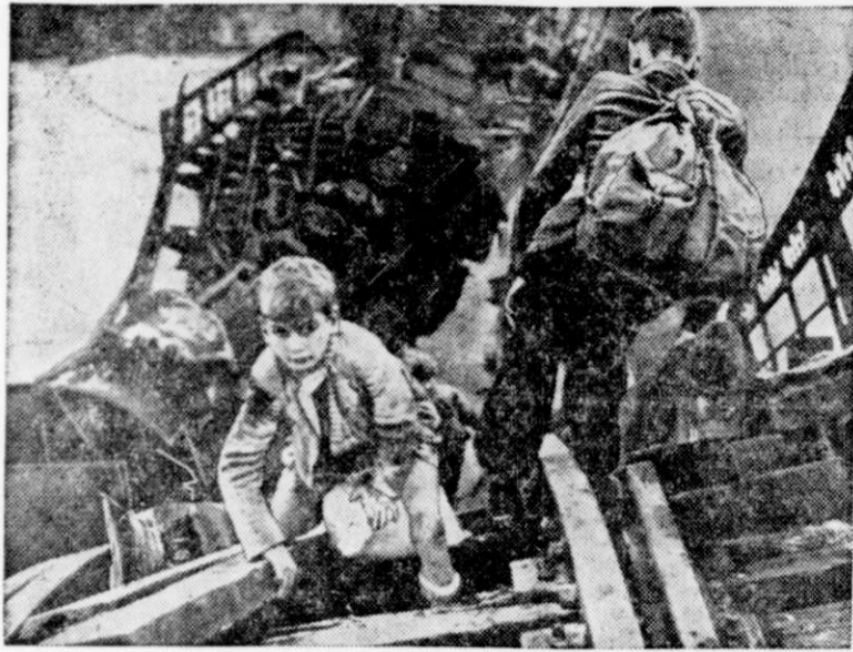
As train lies at bottom of Moselle river after plunging through wrecked bridge, French youth scramble over debris to salvage food from cars.
