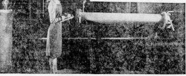
Impregnating apparatus in the Du Pont experimental laboratories is rather simple. The wood is placed in the horizontal cylinder. The overhead tank contains the solution of methylolurea, which flows down and impregnates the fibers of the wood. A vacuum is first created in the cylinder, then pressure.
