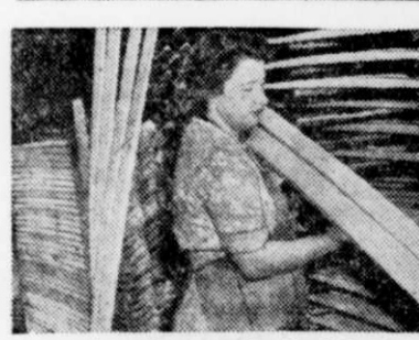
A worker stacks "bedslats" on drying racks. Later they will be waxed. Ski harnesses are not attached by workers but by troopers.
