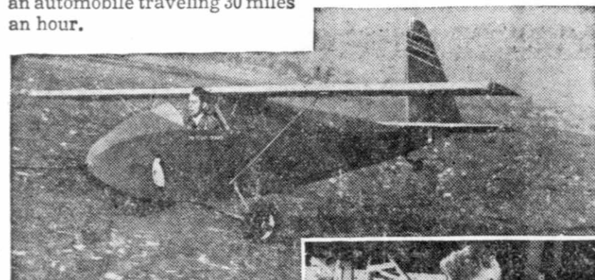
Breaching along behind the tow car, the cadet above tries to prevent the glider's wing tips from scraping the ground. Perfectly controlled, the glider will roll smoothly with tail up and wings level.
