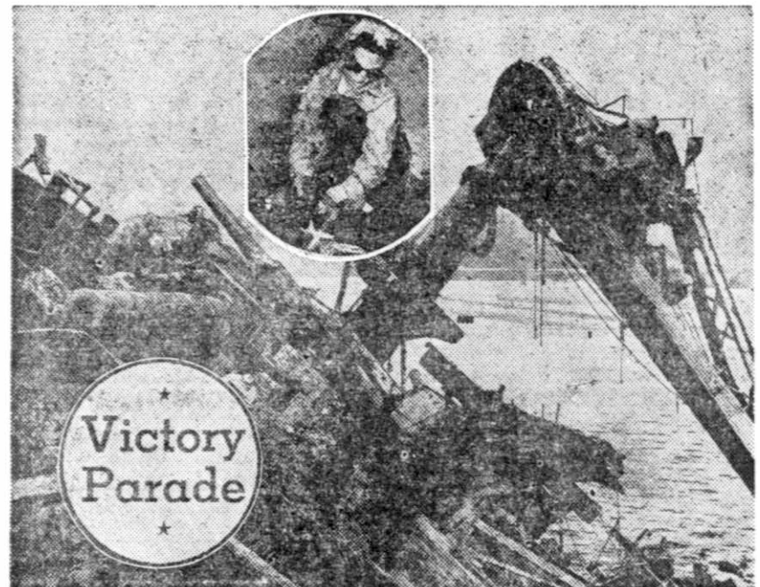
Damage and corrosion to the superstructure of the Oklahoma are quite pronounced in this picture. Inset: Some of the navy shipyard workers are women. Dorothy Waiwaiole, Hawaiian, is shown cutting steel to be shipped back to the mainland.
